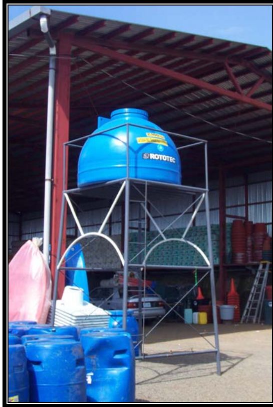
Figure 6 - 7 Elevated Polyethylene Storage Tank
